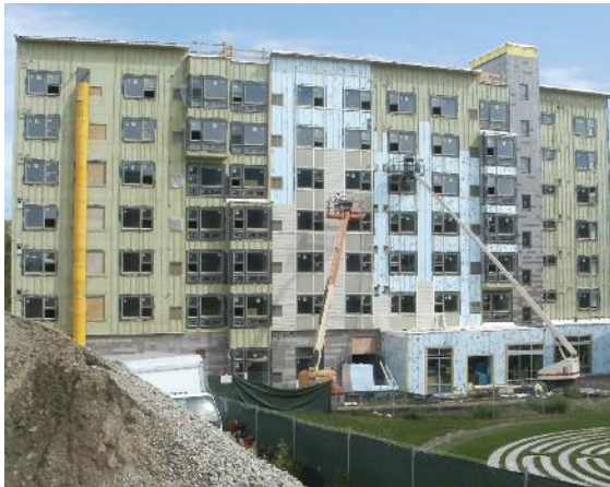
Malkin Construction hard at work
